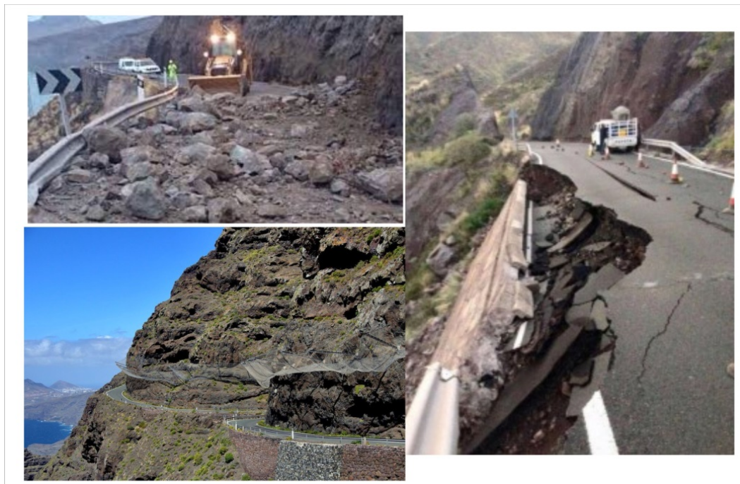
Figure 5: The GC- 200 road between the localities of Agaete and Aldea. It is considered one of the most hazardous roads in Europe. Numerous rockfalls cut the road off every year.
