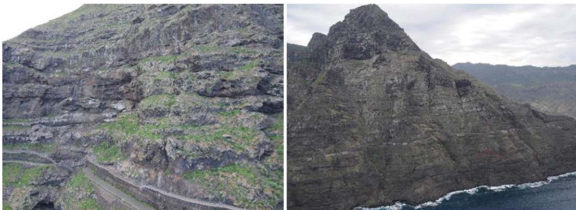
Figure 1: The GC- 200 road between the localities of Agaete and Aldea. It is considered one of the most hazardous roads in Europe. Numerous rockfalls cut the road off every year.
